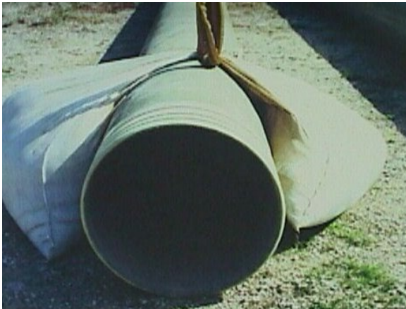
Figure 10: Sandbags on GRP pipes
