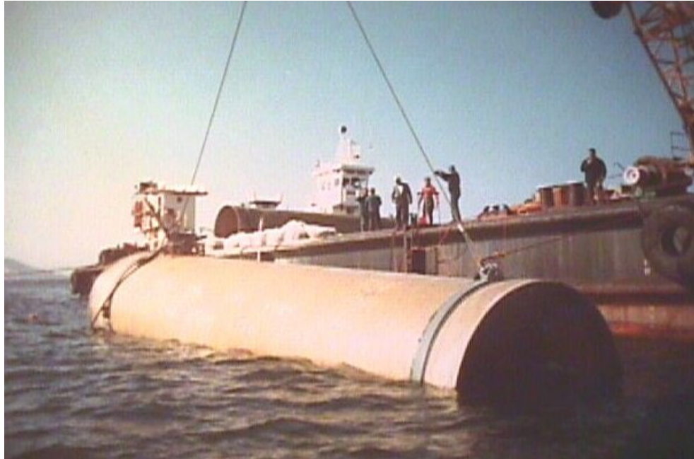
figure 9: Lowering a single pipe section from the pontoon.
