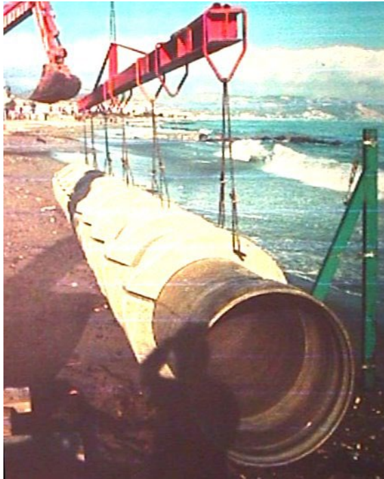
Figure 8: Pre-assembling of the pipeline on the beach.
