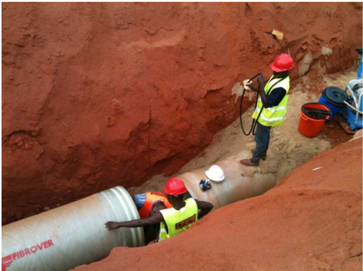
Figure 1: Laying a pipe in the trench.
