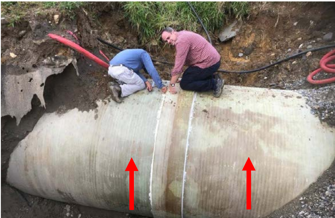
Figure 18: Flotation.
