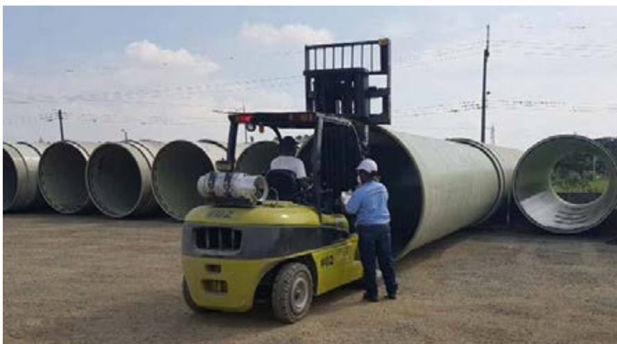
Figure 3: De-nesting with a padded boom.
