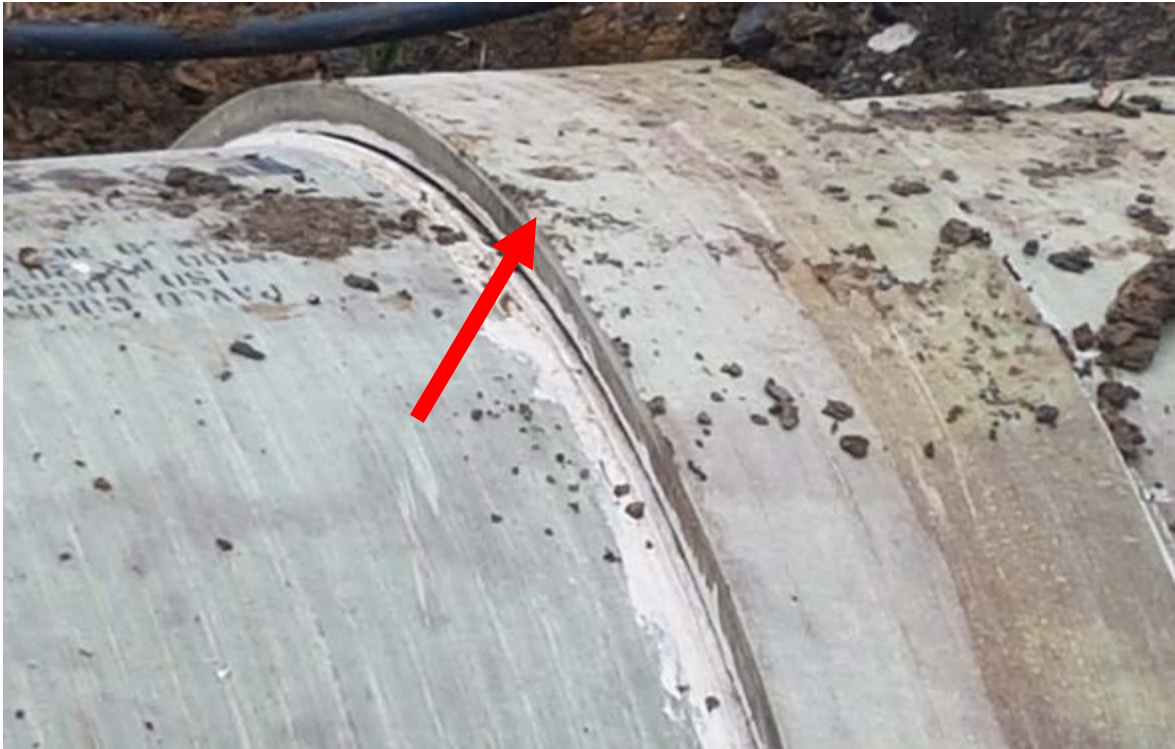
Figure 17: Gap between the pipes, caused by flotation.
