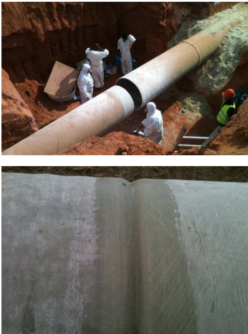
Figure 1: Preparing the surface.
