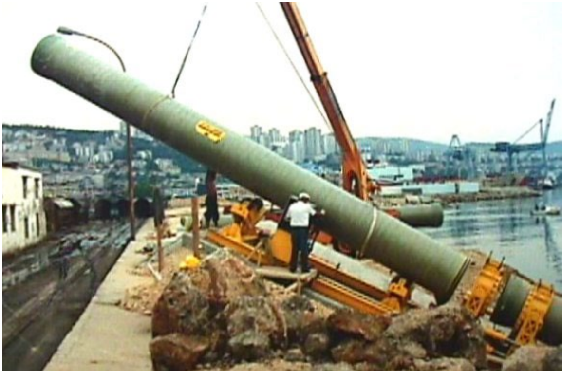
Figure 7: Launching and Jointing machine.
