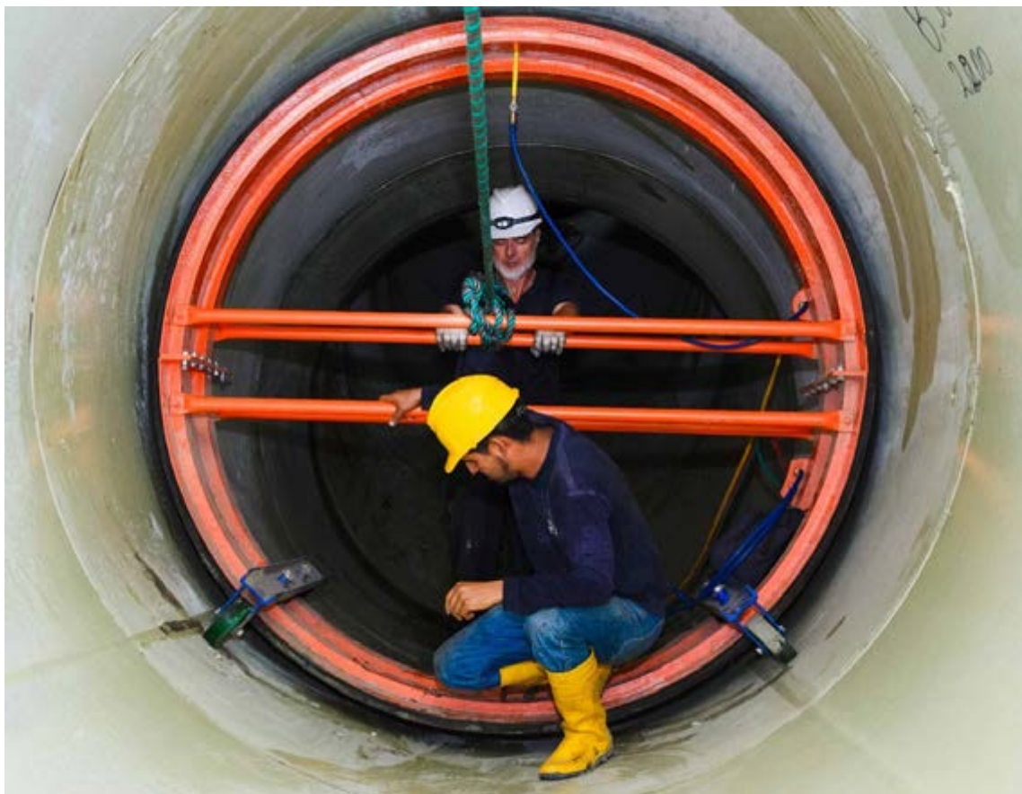
Figure 14: Field joint tester.
