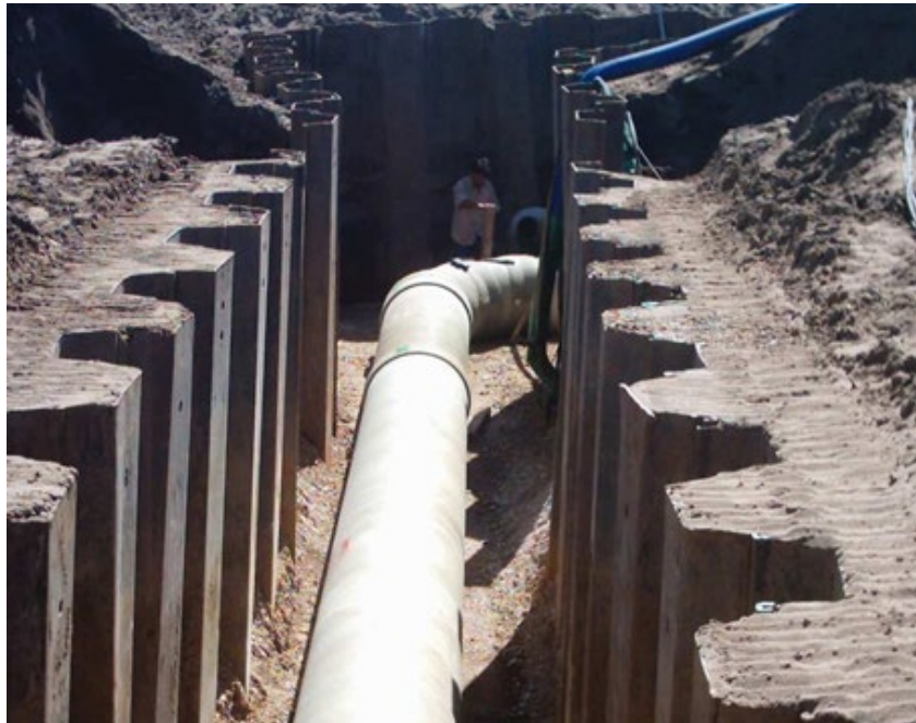
Figure 10: Sheet piles.
