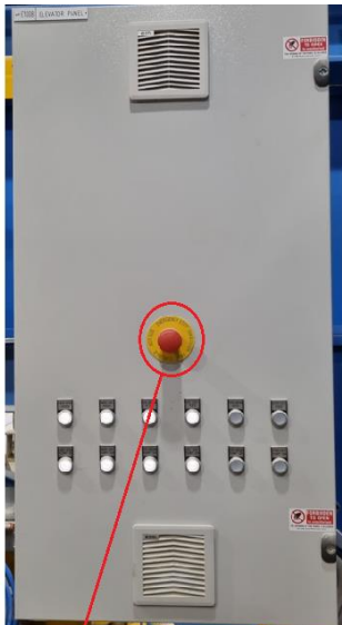
ELEVATOR CONTROL PANEL AND ELECTRIC BOARD EMERGENCY STOP
