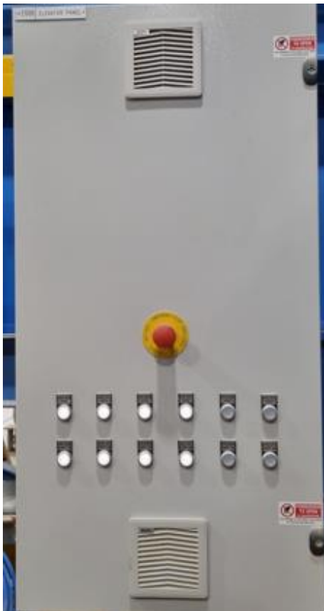
ELEVATOR ELECTRIC BOARD
