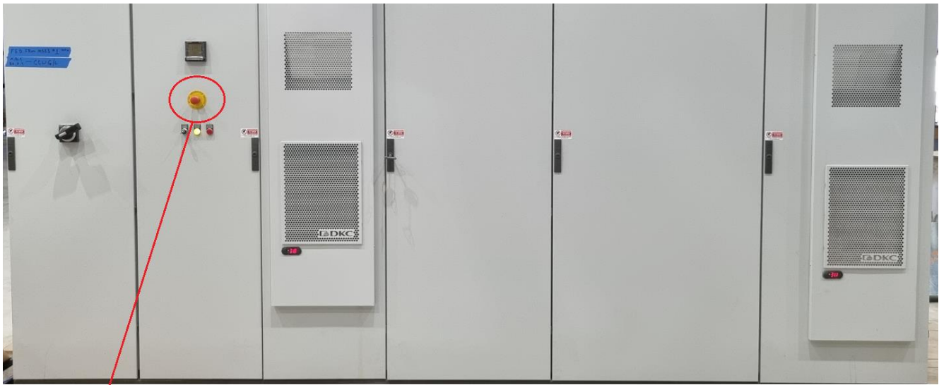
CONTROL PANEL AND MAIN ELECTRIC BOARD EMERGENCY STOP
