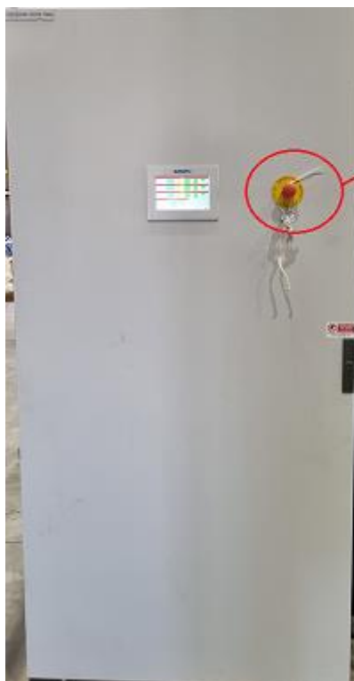
DOSING STATION CONTROL PANEL AND ELECTRIC BOARD EMERGENCY STOP
